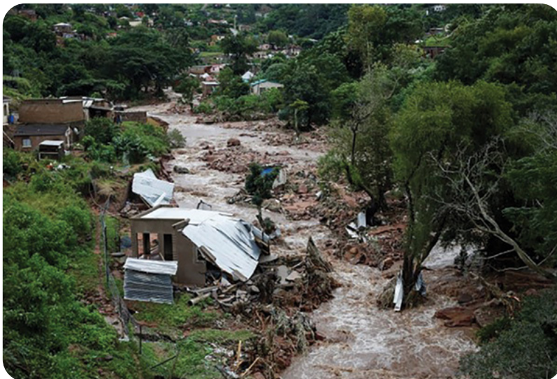
A view of flood-damaged homes in KwaNdengezi, Durban .Photo credit Rogan Ward,Reuters.
