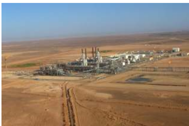
Kechba gas plant, Algeria
