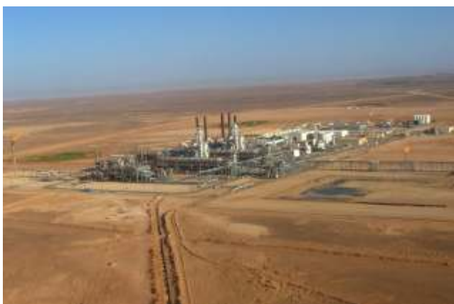
Kechba gas plant, Algeria
